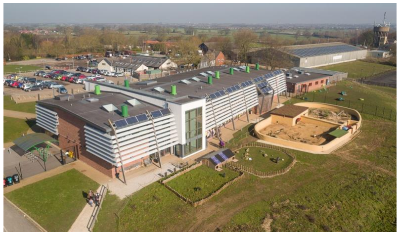
Figure 6 – the roof of Askham Bryan animal management centre (aspect 4, 2015)
